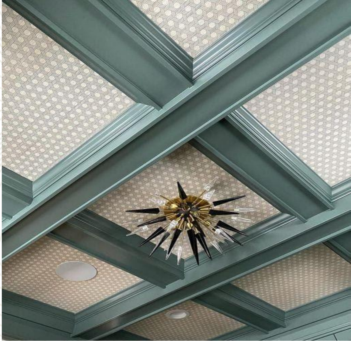
Wooden Coffered Ceiling
